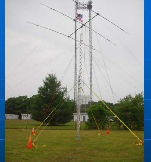
Beam antennas will be hooked up to a triplexer allowing three stations to use one tri-band antenna
